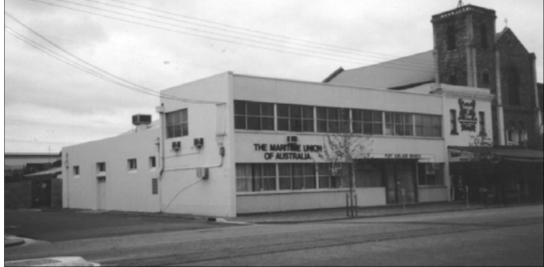
Doug's Shipping and Forwarding Business - The building on Vincent Street today
